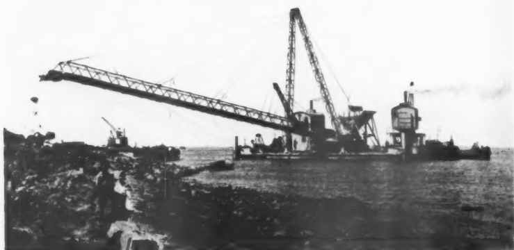
Phot. W. Verkerk, Amsterdam Discharging boulder clay by travelling belt
